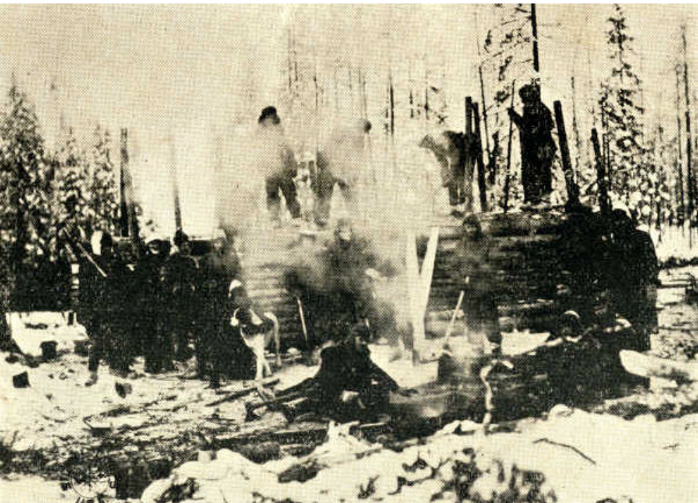
U. S. OFFICIAL PHOTO Building a Blockhouse
